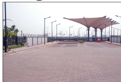
Concrete roads and Gate House
